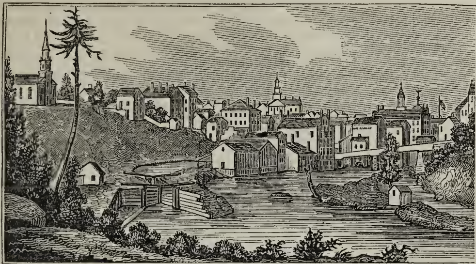
East view of Seneca Falls village.
